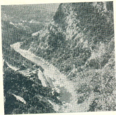
MAHATMA GANDHI POWER HOUSE
