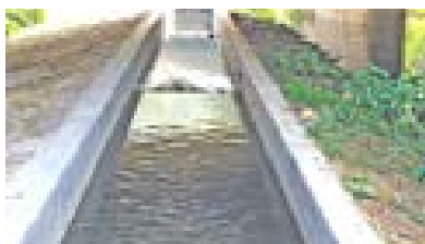
1. COLLECTION AND SCREENING [UNDERBRIDGE] Area: 600 sqmts [Depth: 1 m appx = 600 cumts appx] Duration: 24-48 hrs
