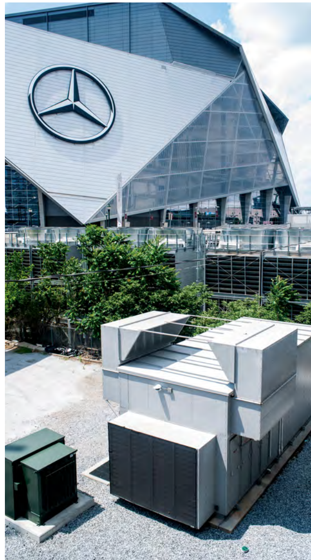
The Vapor IO Kinetic Edge modular data center site outside of Atlanta's Mercedes-Benz Stadium is about the size of a shipping container and can support up to 24 separate “tenants.”
