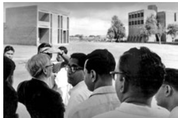
1968 pictures of the IIM-Ahmedabad [IIM-A] under construction show no signs of the city
