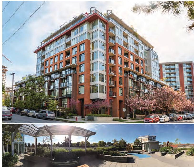
The fifth-floor community space at the Social condominium building in Vancouver is a gathering spot for families. Parents can socialize and watch their kids as they play.
