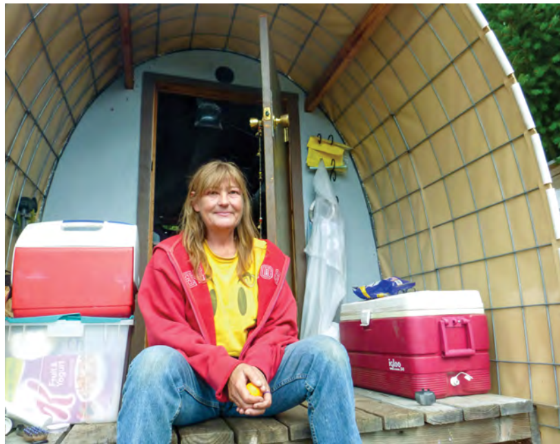
The Conestoga Hut Micro-Shelter is one quick, temporary shelter option, offering 60 square feet of interior space and an insulated floor, walls, and roof.
